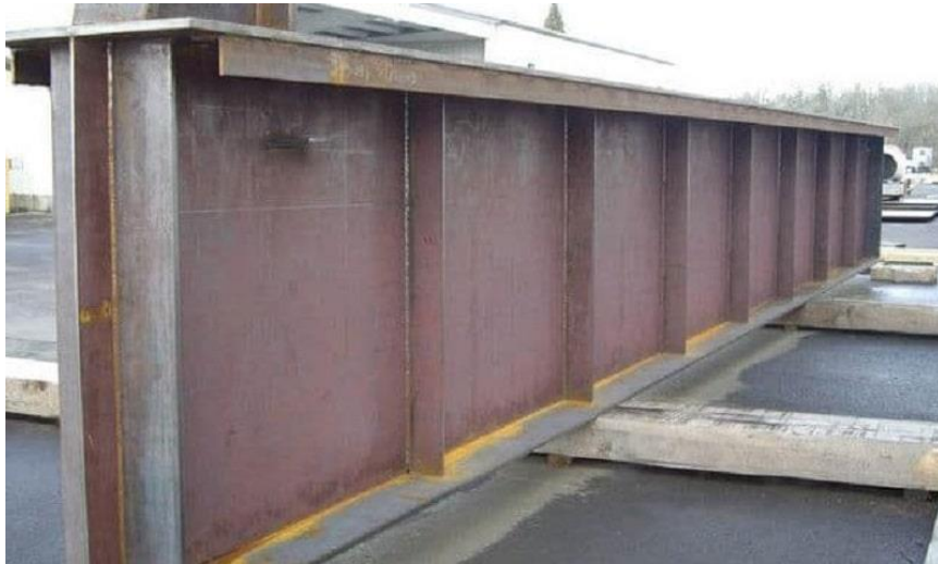
Fig.2 Plate Girder – Typical Built-up beam section along with Stiffeners to resist heavy load in bridges
