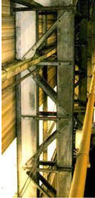
Fig.1 Typical laced column
