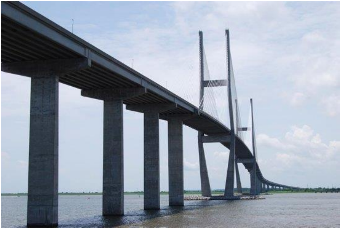
Fig.5 Continuous Beam - Bridge
