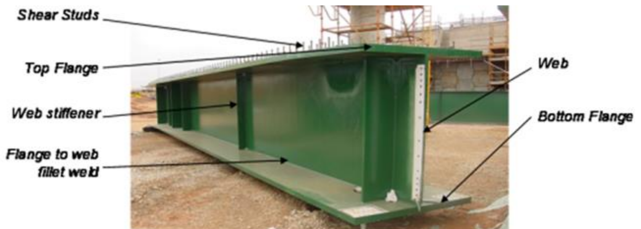
Fig.3 Plate Girder – Components
