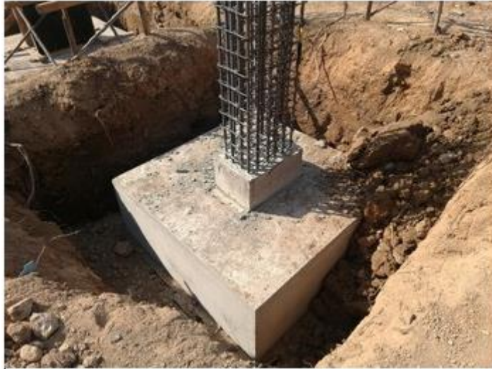
Fig.2 Typical image of isolated footing
