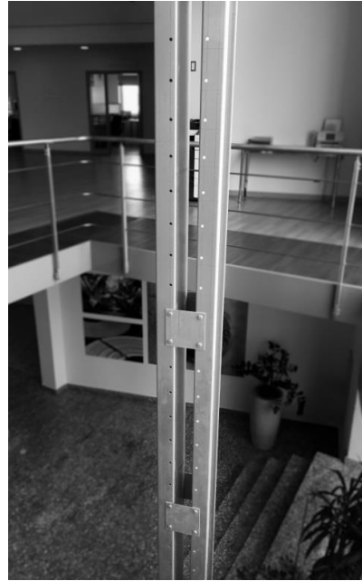
Fig.2 Typical batten column
