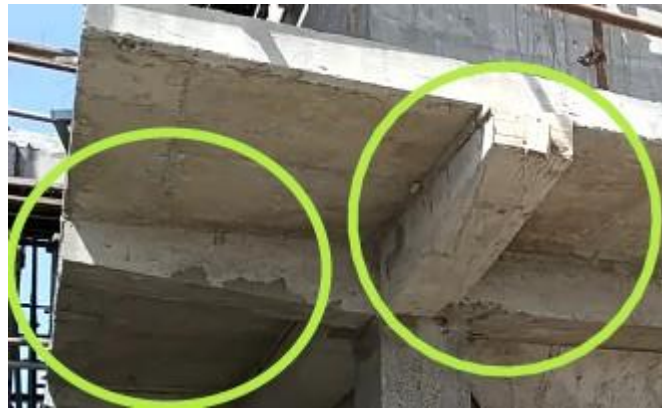
Fig.1. Cantilever Beam – Building Construction
